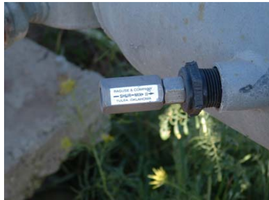
Injection Line Check Valve
