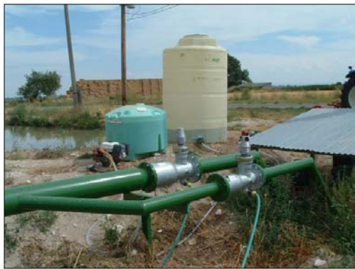
Chemigation Valves with Vacuum Relief Valves, Low Pressure Drains and Hoses installed.
